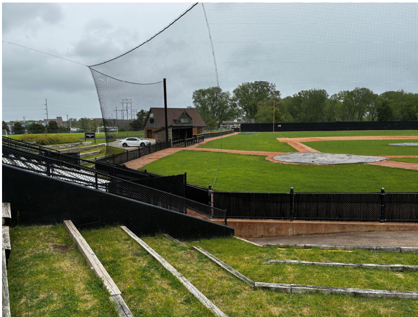
From bleachers looking east to construction access
