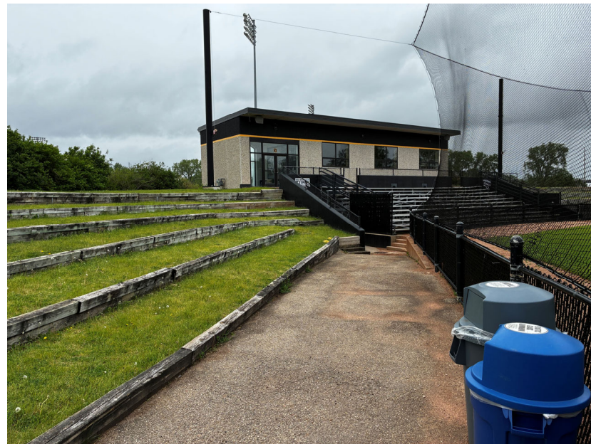
Looking north to main bleachers
